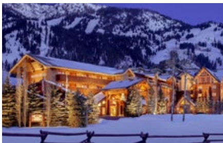
SNAKE RIVER LODGE 4★ ROOMS, SUITES, CONDOS AT BASE
